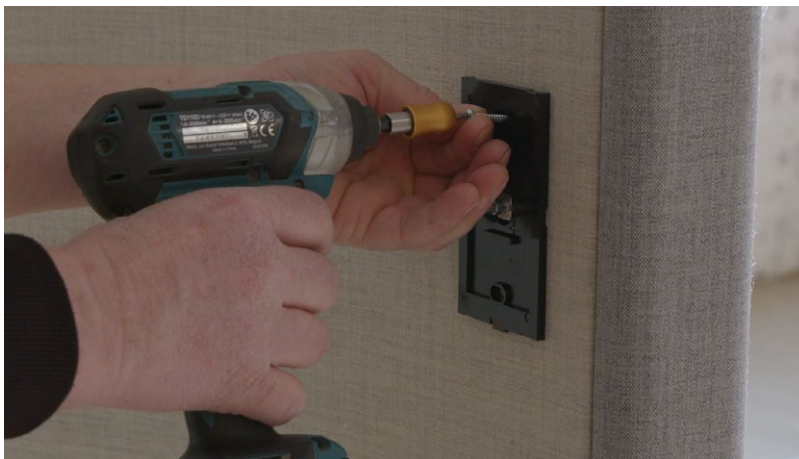
Insert the dimmer to the screen and screw it with wooden screws.
